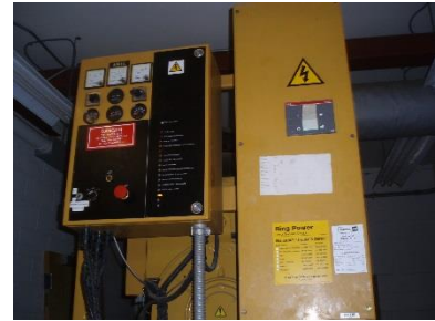
Figure 2-3. Electrical Vault Backup Generator
