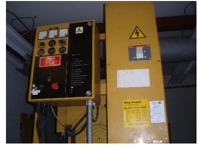
Figure 2-3. Electrical Vault Backup Generator
